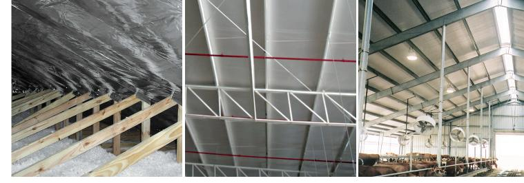
**Foil/Foil** Increases home comfort in between conditioned and unconditioned spaces. White/Foil May be used as a condensation blanket in well ventilated buildings.
