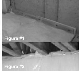
of the wall depending on specific construction details. Trim any excess insulation for a neat appearance. Pull the release paper from the factory applied double stick tape. Overlap this 6" facing tab and adhere to the adjacent blanket.
